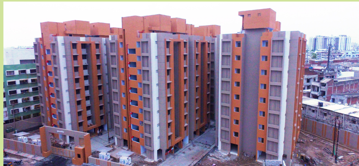
Houses constructed under AHP, Surat, Gujarat
