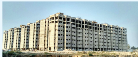
Completed project under In-Situ Slum Redevelopment of PMAY(U) in Baroda, Gujarat
