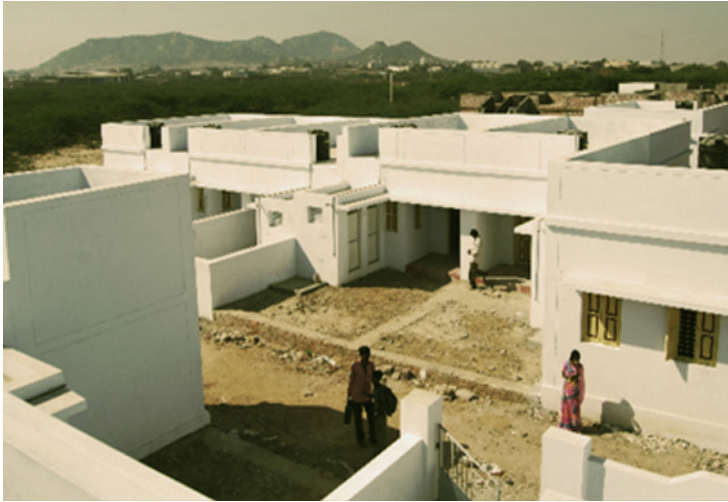
Housing structures before completion at Ramdev Nagar slum rehabilitation site.
