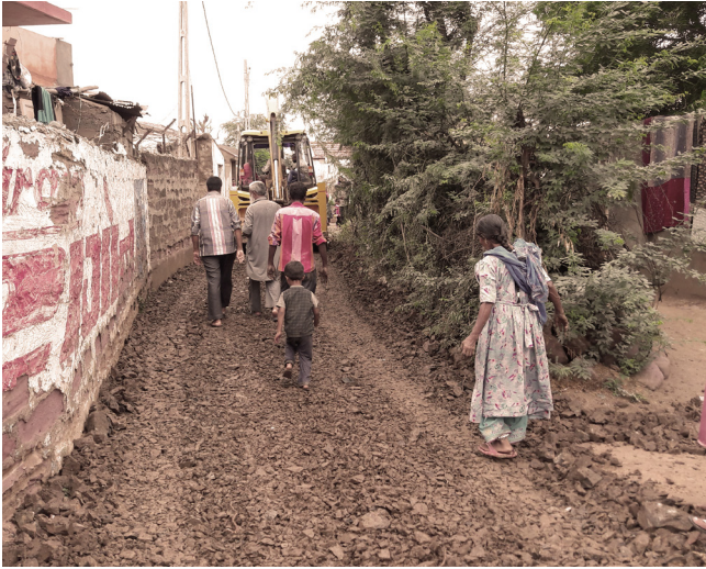
Road repairing work is on going under supervision of ward committee in Shaikh Falia in Ward no. 2
