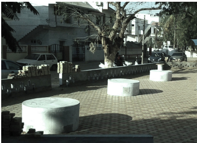
Ground water recharge points at Jublee colony
