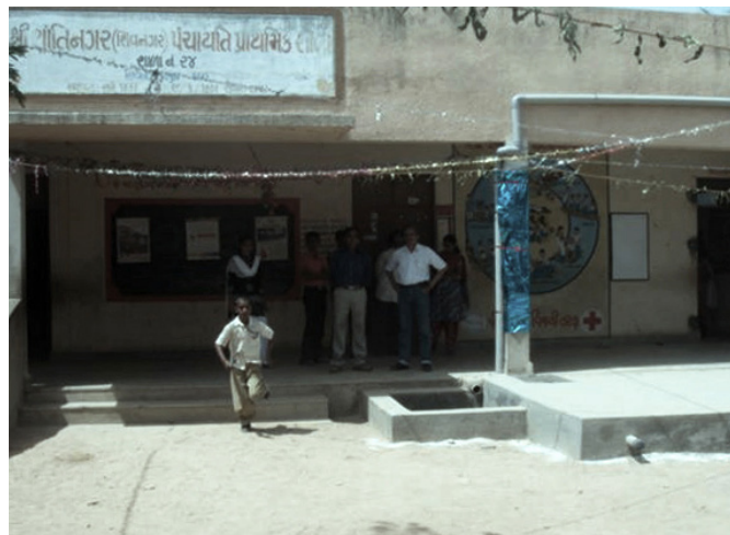
Roof rain water harvesting system installed in a primary school building
