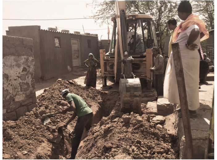
On going excavation work to lay down water supply pipeline in Bhagatwadi area in ward no. 3
